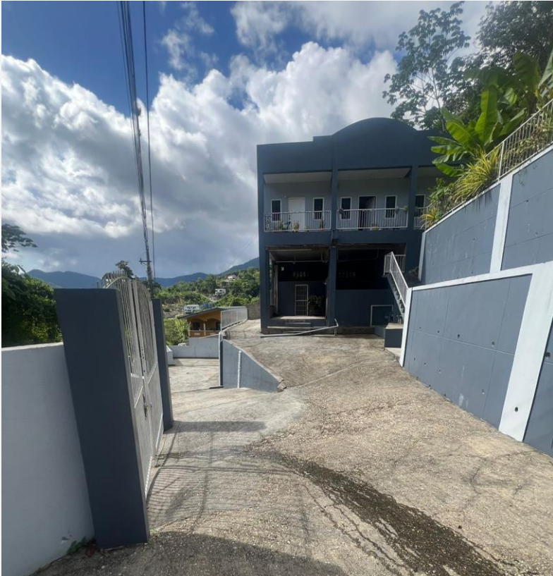
View of Building Frontage
